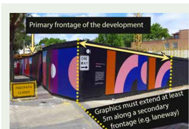
Figure 6.7: For a corner site adjoining a laneway the installation of graphics on the secondary road (laneway with a width not exceeding 6 metres) must extend a distance of at least 5 metres from the primary road hoarding frontage as indicated (refer to 'Note 2' in Table 1 ) and the remainder of the hoarding must be painted flat black.
