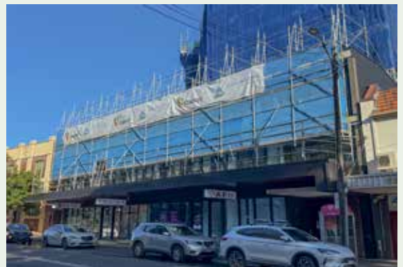
Figure 4.9: Example of scaffolding supported on a street awning. Note that the City will only consider permitting this in limited circumstances (refer to 4.6.7(d) ).
