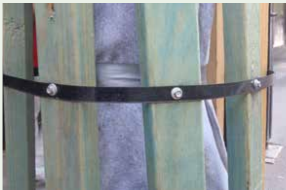
Figure 3.64: Tree trunks must be fully protected prior to the erection of the temporary structure and unless specifically directed by the City, remain in place for the full duration of the development or work. Timber battens protecting trunks must be securely fixed using flexible steel or durable fabric banding and the band-ends finished neatly to avoid protruding sharp edges. The City's preference is for fabric strapping to be used (securely fixed and maintained tautly).
