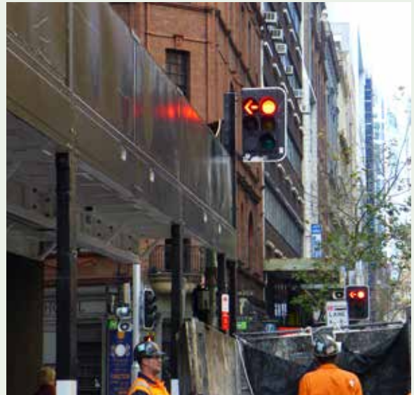
Figure 3.29: The design of temporary structures must maintain viewlines to traffic signals. In cases where signals need to be modified and/or temporarily repositioned the approval of Transport for NSW must be obtained.
