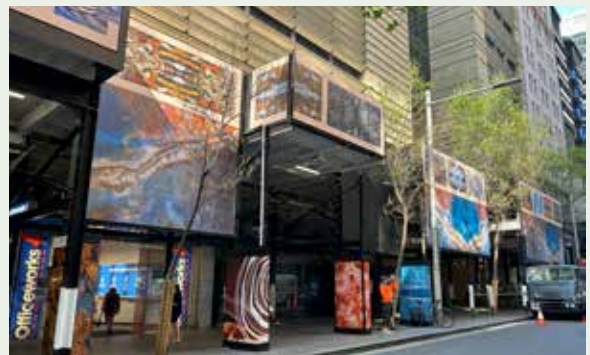
Figure 3.28: Some forms of bracing elements must be screened from view when located on the kerbside and painted black below the deck (see 3.8.8 ).
