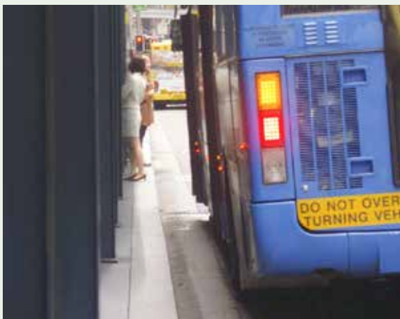
Figure 3.18: The positioning of hoarding columns along the kerb and at bus-stops (passenger loading and unloading areas) must be given special design consideration (see 2.8.4(f) for details).
