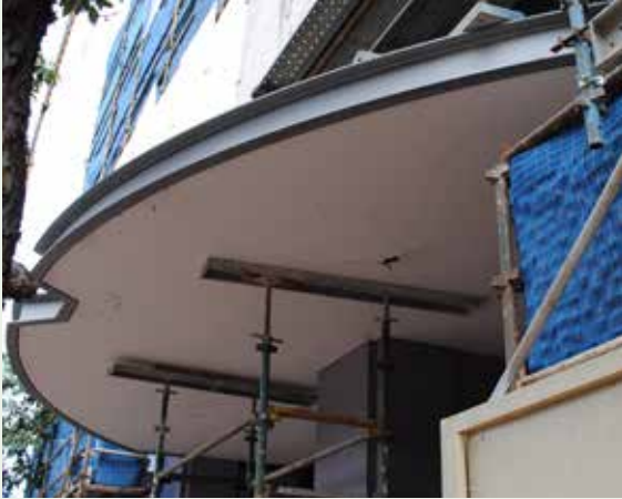
Figure 4.10: Under some circumstances the City will allow scaffolding to be installed on a street awning if satisfactorily supported from the footway below. These designs must be fully engineered and a detailed assessment made of the structural condition and adequacy of the existing awning. This must be fully documented and certified and included with an application (see 2.8 for certification requirements).
