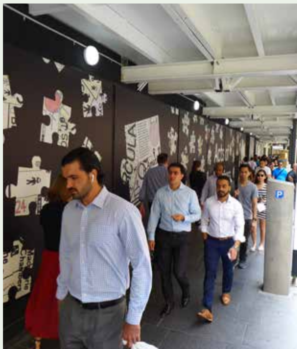
Figure 3.21: An assessment of the locality (street infrastructure and footway width) and pedestrian densities must be made as part of the hoarding design process. Site fence and column encroachments must be minimised to maintain safe, convenient and accessible passage of pedestrians, delivery workers and users of wheelchairs and mobility scooters.
