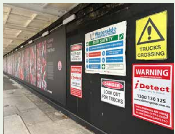
Figure 6.17: All mandatory signage, other than minor caution signage and parking control signage, must be displayed at the ends of hoarding fences or next to access doors. Signage must not be placed over graphics.
