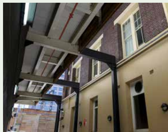
Figure 3.52(a): A Type-B hoarding showing a section of open deck (located away from the worksite) to maintain solar access to the building opposite. Proponents must consult with affected property owners as part of the hoarding design process. The placement of sheds on decks in these circumstances is discouraged. Refer to 5.5 for further requirements.*
