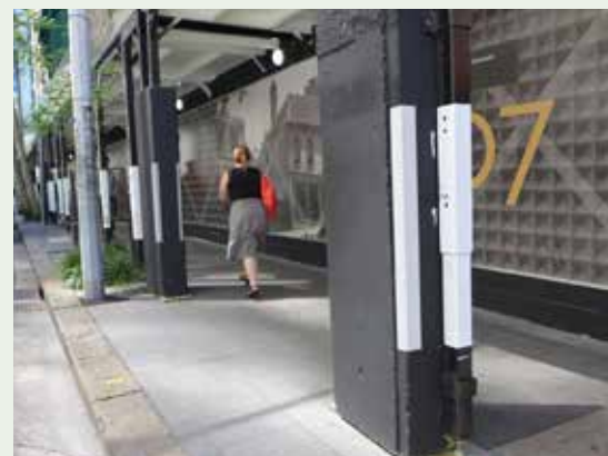
Figure 3.22: Where ground or surface conditions have insufficient bearing capacity to support a temporary structure the City will consider allowing recessed steel plates within the footway subsurface to provide support. Concrete footings may also be considered (see 3.8.5 ). The area surrounding recessed plate/s (or on top of the plate) must be backfilled and evenly finished with material specified and approved by the City . A separate approval ( road opening permit) must be obtained prior to undertaking any work.
