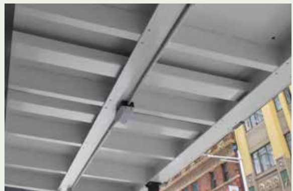
Figure 3.62: All wiring for lighting systems must be placed within conduits complying with the applicable wiring standards. Conduits on site fences must be painted to match the background colour surface (black). Where installed on the underside of the deck, conduits must be white or grey.
