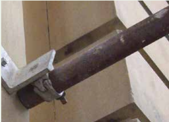
Figure 4.3: Scaffold fixings to heritage-listed buildings should be avoided but where necessary, comply with the provisions in 4.4.2 .
