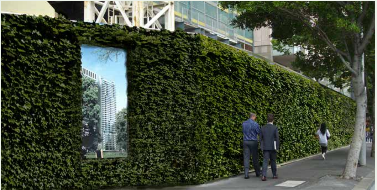
Figure 6.1: Finishing site fences and hoarding fascias with a ‘green wall’ installation is an innovative and attractive way to mask development sites in prominent locations and improve streetscape amenity. Where approval is given specific conditions will apply including minimum ongoing maintenance requirements.
